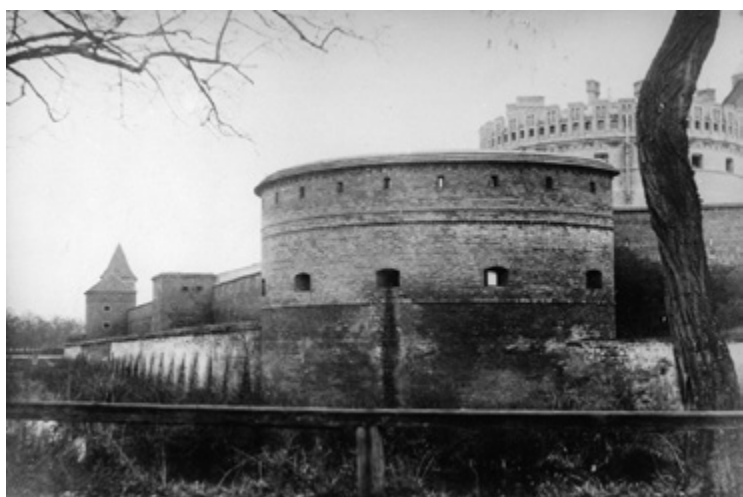
Ill. 20. Toruń. View of the medieval city walls from the north-west side, in the background – the prison building from 1865, 1888 (State Archives in Toruń)
