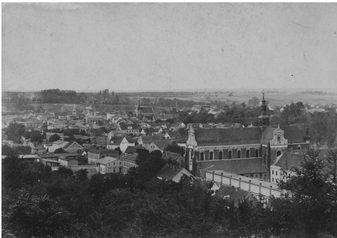
3. Koronowo. The general view from the southern west, c. 1895, (photo)
