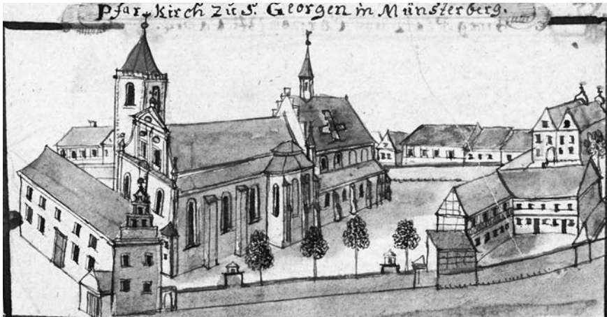
6. F.B. Werner, St. George parish church, overall view, 1762–1771
