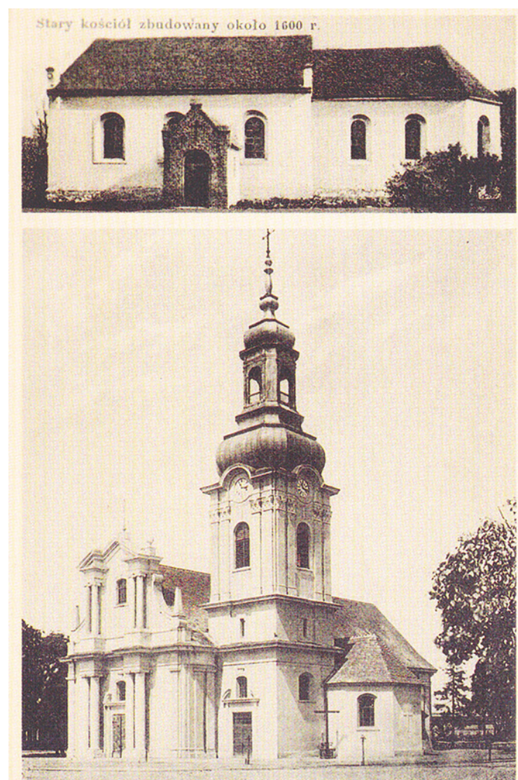
Fig. 1. Fordon. Parish church of St. Nicholas before and after rebuilding, around 1935. the top – the view from the south before the reconstruction of the church; the bottom – the view from the southeast after the reconstruction by Stefan Cybichowski, an architect, in the years 1926–1930 (postcard, published by L. Ziolkowski, Fordon, after: Bydgoskie świątynie na dawnych widokówkach z kolekcji Wojciecha Banacha , Bydgoszcz 1997, no. 12)
